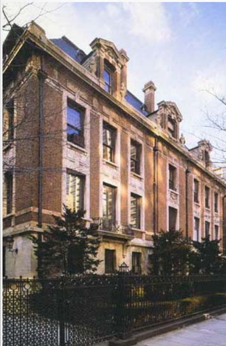
The front driveway at the former Playboy mansion, 1340 N. State Pkwy., is to be turned into a garden.
